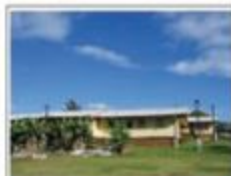
Hawaii Public Housing Authority
